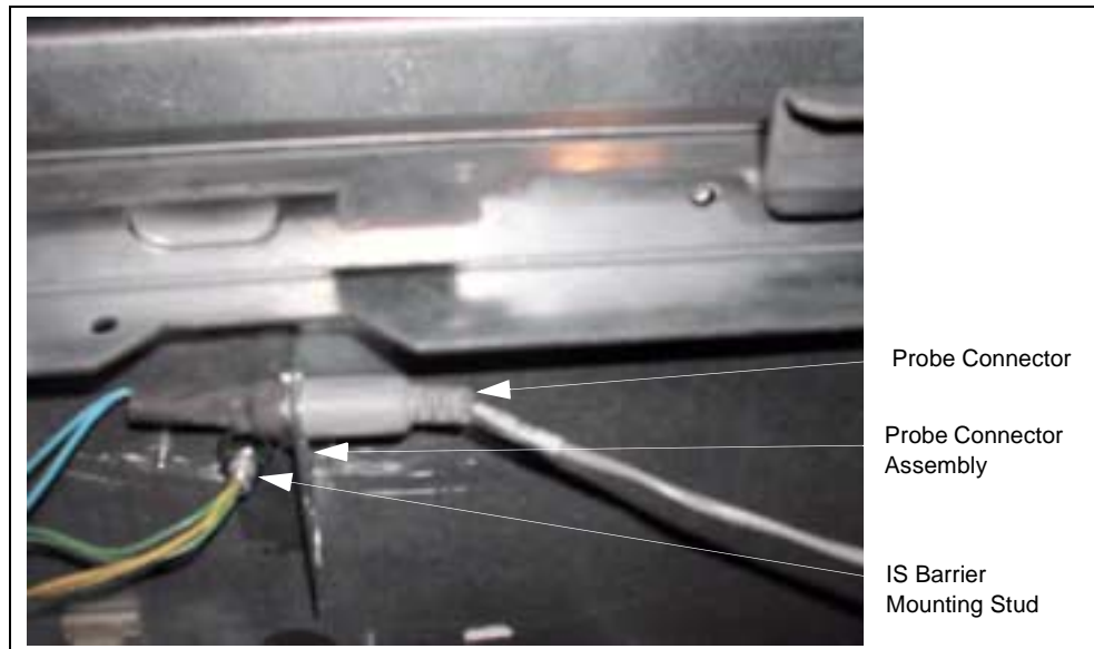
Figure 5: Probe Connector Assembly and IS Barrier Stud Mounting (Underneath Shelf)
